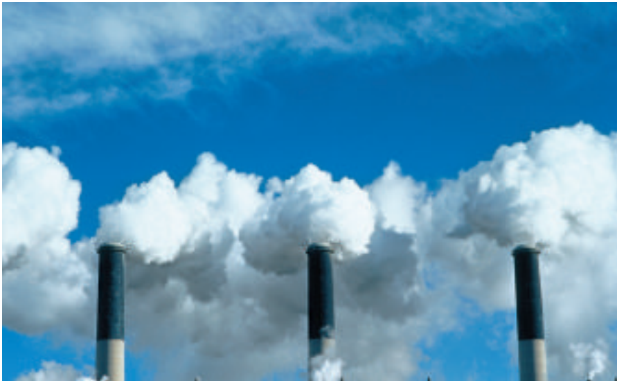
■ Figure 20-12 The fly ash being released by these smokestacks is a by-product of burning coal. Static-electricity precipitators can be used to reduce fly ash emissions.
