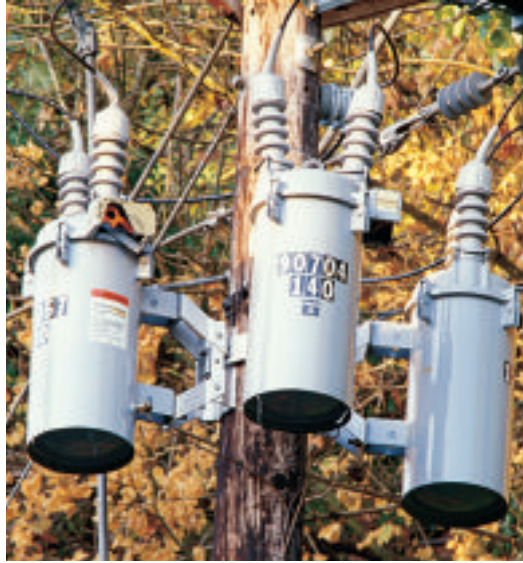
■ Figure 26-11 In a transformer, the amplified oscillation from the secondary coil is in resonance with the coil-and-capacitor circuit and keeps the oscillations going.
